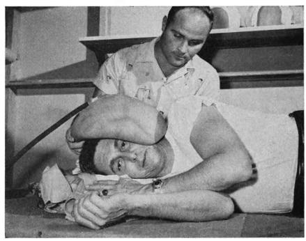
**CUSTOM FITTING** was essential for every inch of Crossfield's space uniform. Here, he has a mold made of his head for helmet he wears in X-15.
